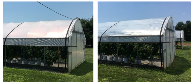
Figure 3. The plastic cover on the left is KoolLite Plus, which is a diffusing plastic that blocks some wavelengths from entering the tunnel, and the one on the right is Tufflite IV, a clear plastic with high light transmission. Note the differences in how light is reflected and what you can see through the plastic.
